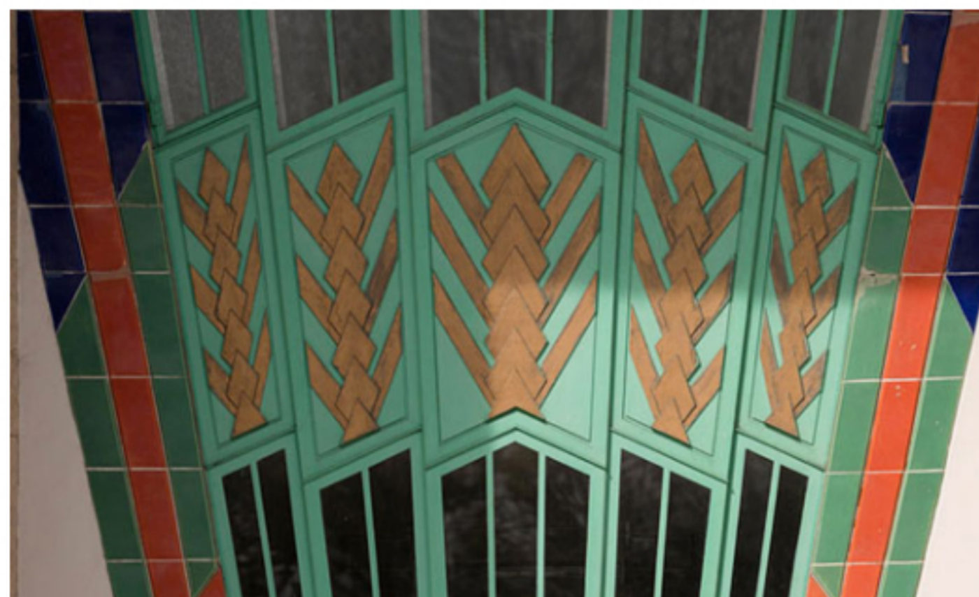
Apartments in the 1930s Wallis, Gilbert and Partners-designed art deco Hoover Building in Perivale, west London
