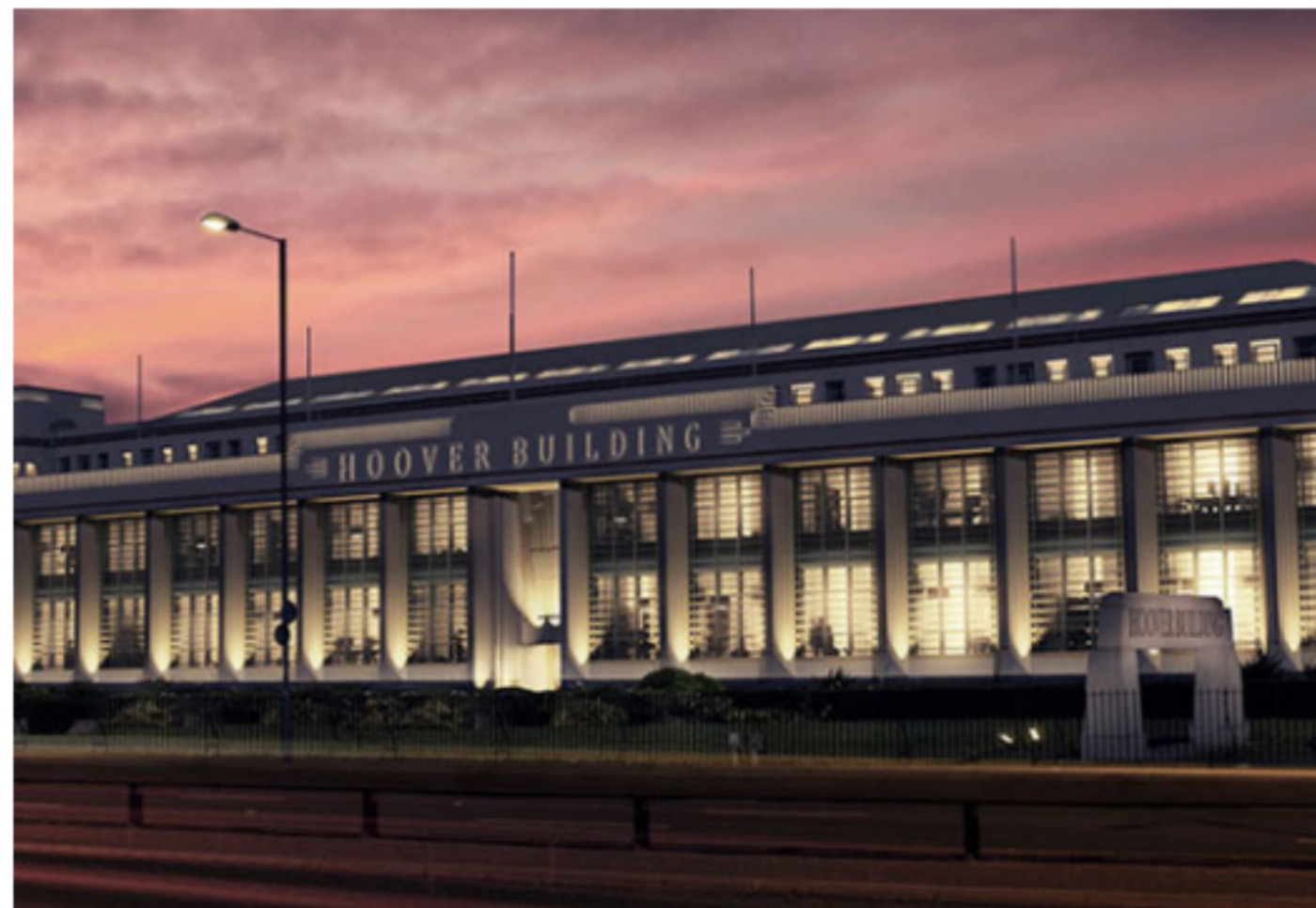
Apartments in the 1930s Wallis, Gilbert and Partners-designed art deco Hoover Building in Perivale, west London
