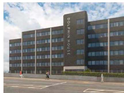
DOLPHIN HOUSE Windmill Road, Sunbury TW16 7HE
